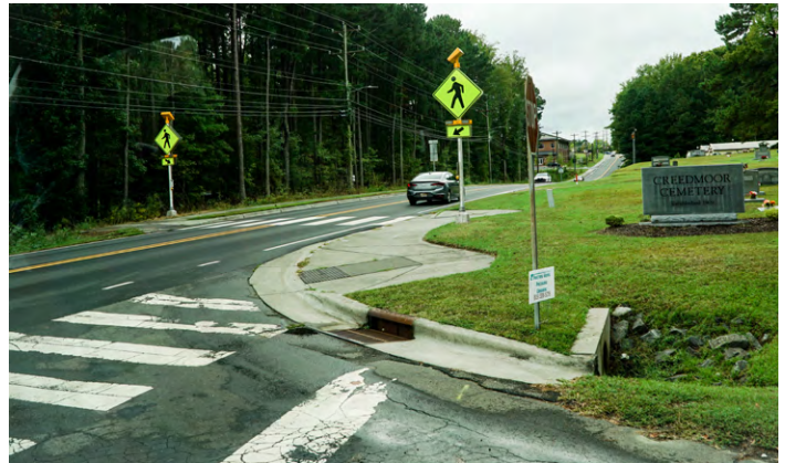
Pedestrian crossing on NC 56.
