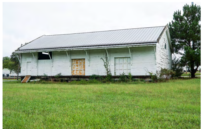
Old railroad depot (Source: City of Creedmoor)
