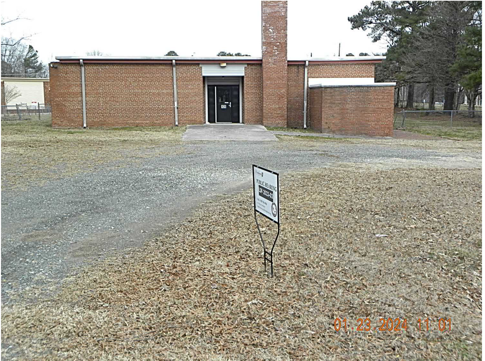
109 Park Ave - Posted in front of 109 Park Ave : Img 2
